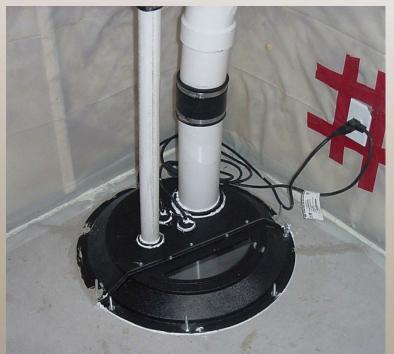
Sealed sump pit lids are available in building supply stores. In many cases, installing a sealed sump lid is the most cost-effective radon control measure.
